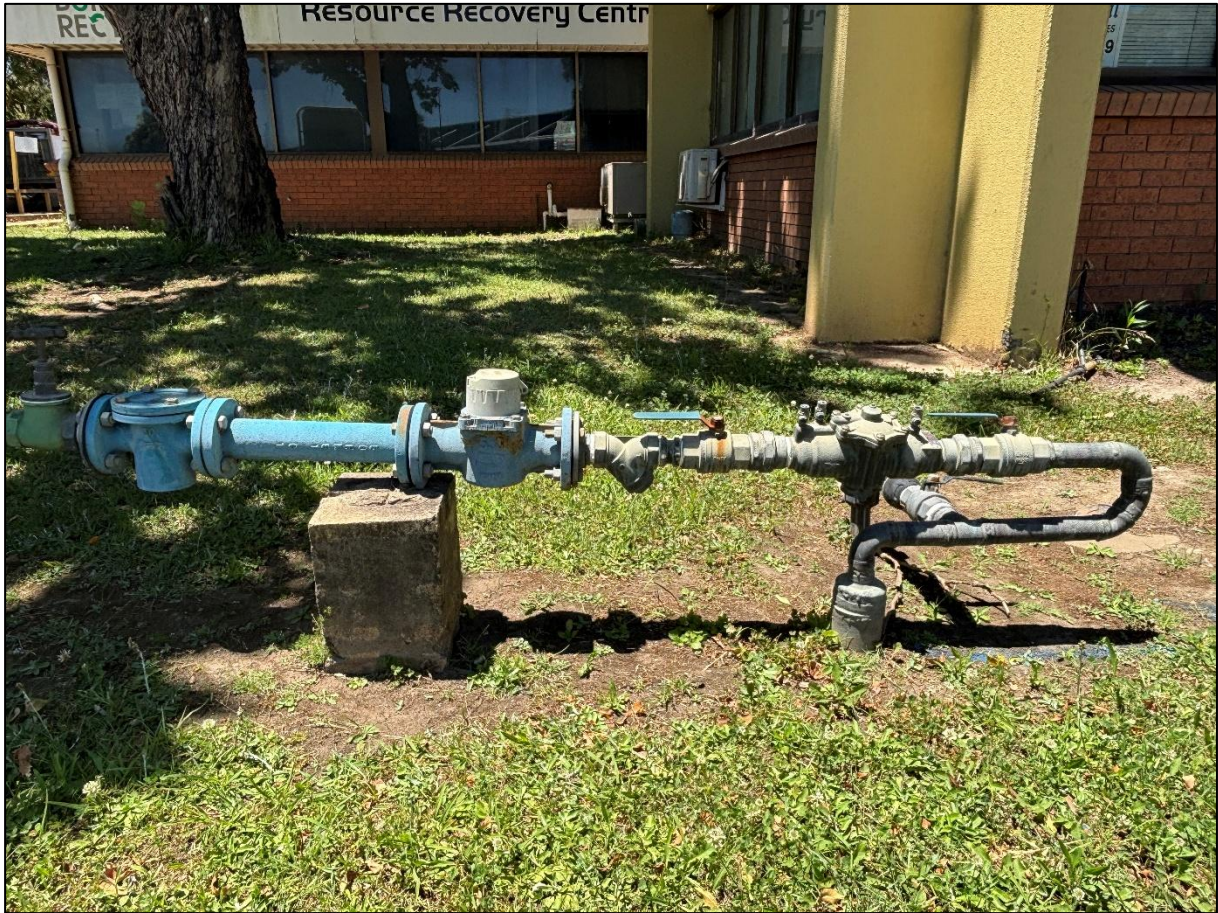
Figure 5 – Site Photo showing the water meter and the two stop valves for the watermain within the site (Extract from Site Photos)
